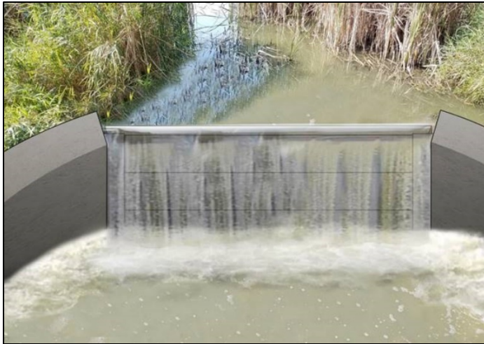
Figure 30 - Outlet Structure Modifications
